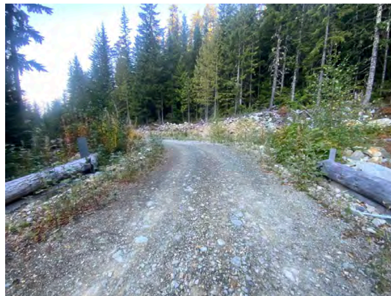
Approach from Right Bank when facing downstream
